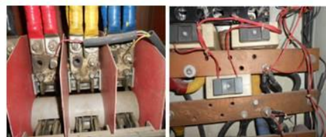
Connections without lugs
